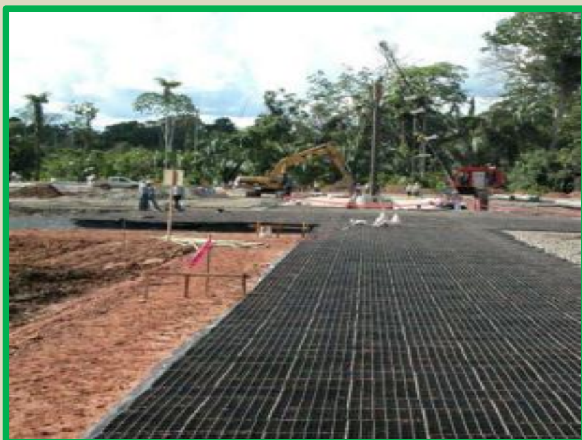
Remote areas runway construction using GeoWeb matting
