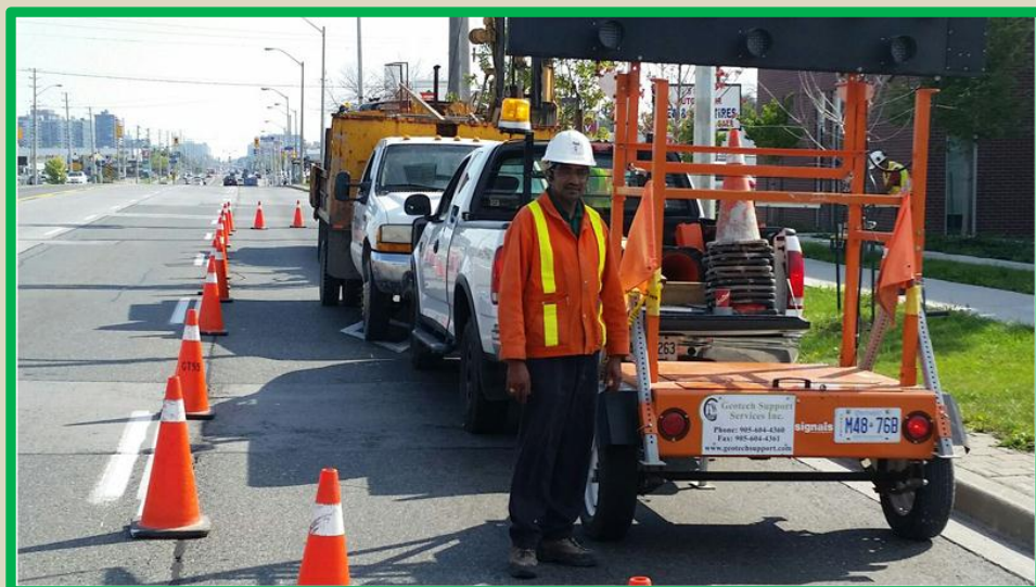
Working safely on busy roadways
