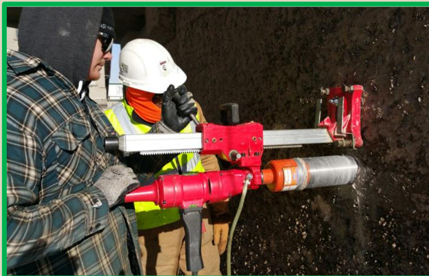
Extracting samples of failed concrete for analysis
