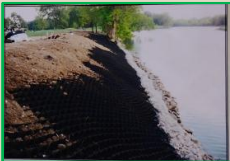
Stabilizing conservancy dams
